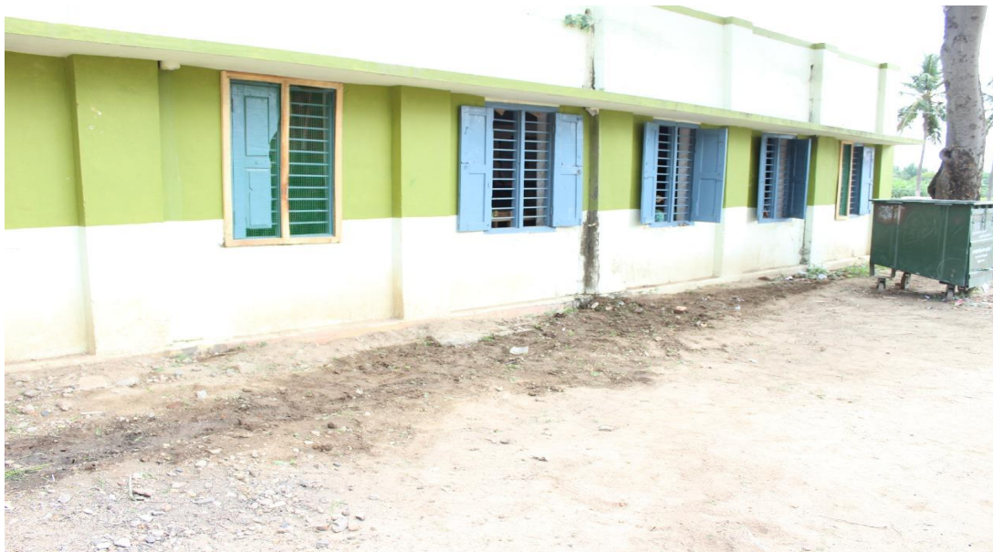
NSS Volunteers of Priyadarshini Engineering College, Vaniyambadi organize cleaning of streets and back alleys in Yelagiri Village
